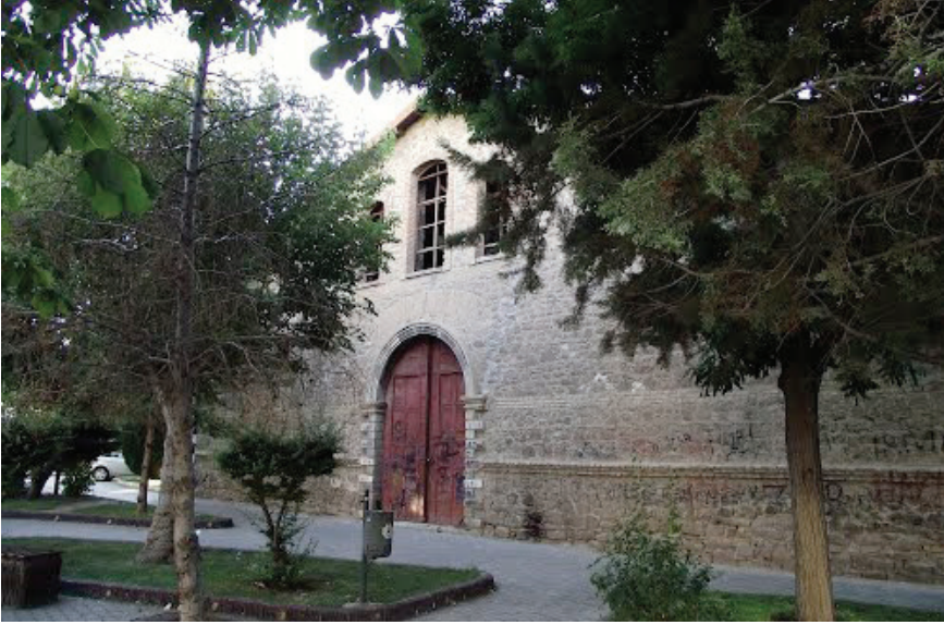
Figure 1. Tantavi Depot Building (Source: Google Earth)
